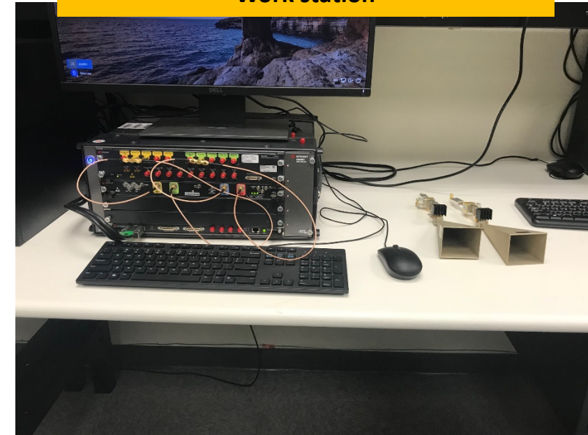
High Data-rate Direct RF Sampling MIMO Work station
